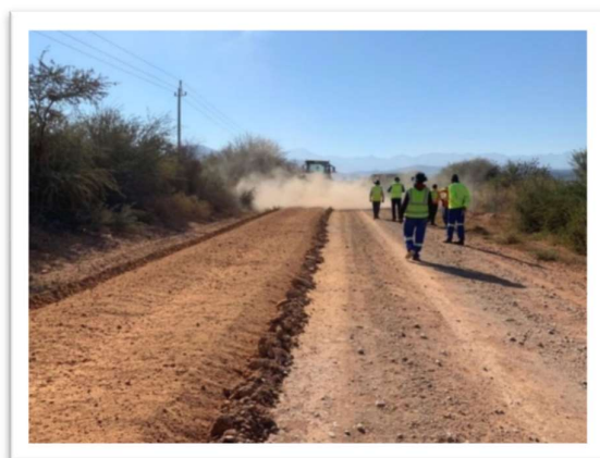
Picture 5-4: Processing the in-situ subgrade using an in-line crusher
