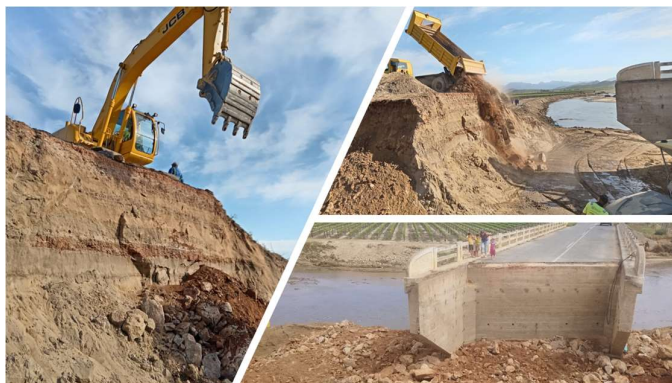
Figure 4-58: Damage caused by September 2023 flooding to MR00290 - Access road to McGregor
