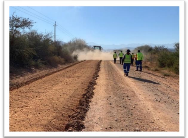
Picture 5-4: Processing the in-situ subgrade using an in-line crusher
